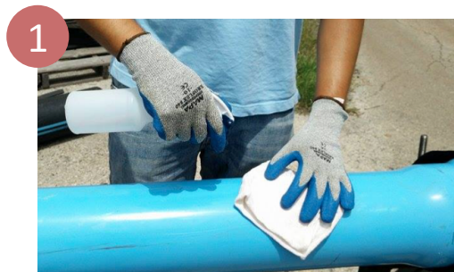
1 Thoroughly clean the pipe where the clamp will be installed.
