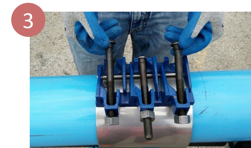
3 Tuck the gasket flap in place, close the bolt lug, engage the centermost bolt(s) and finger tighten. NOTE: using the palm of your hand, squeeze the end of the clamp fingers and the top of the stud lug to bring stud bolt and fingers parallel.
