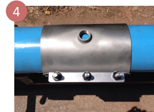
4 Rotate the clamp to flatten the tapered-end of the gasket, and position the bolts and nuts for convenient tightening. Check the reference mark (if used).
