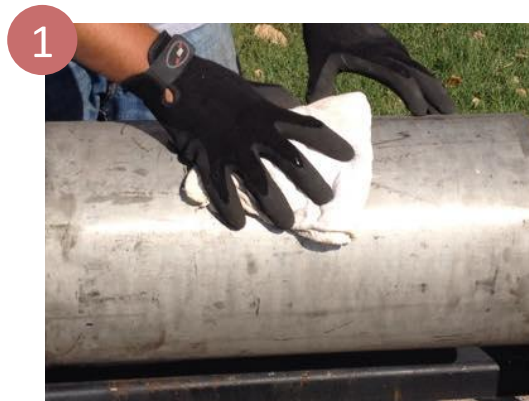
1 Thoroughly clean the pipe where the clamp will be installed.
