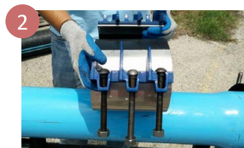
2 Loosen nuts to the end of the stud bolt, and place the clamp around the pipe centered over the break or damage area with the gasket flap at the top.
