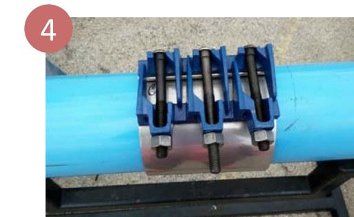
4 Rotate the clamp to flatten the tapered-end of the gasket, and position the bolts and nuts for convenient tightening. Check the reference mark (if used).
