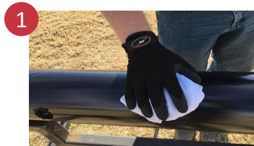
1 Thoroughly clean the pipe where the clamp will be installed.
