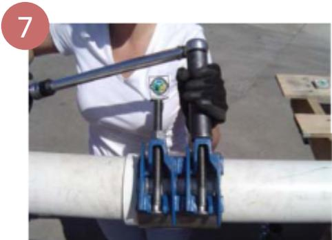
Tighten nuts until clamp is tight or leak is stopped (approximately 70ft-lb of torque).
