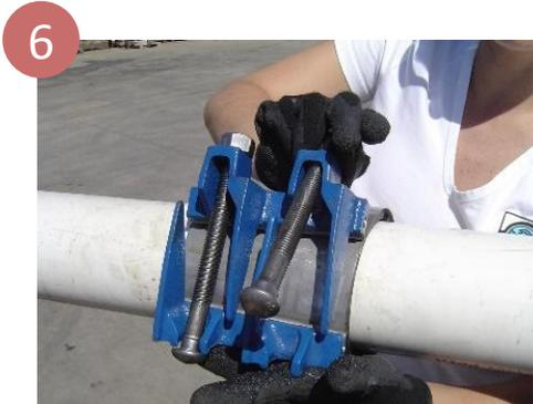
Once the clamp is in the right position, fit the bolts head on the hook of the lug and start tightening the nut by hand.
