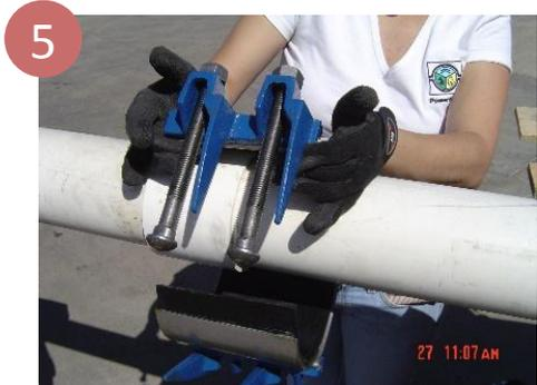
Send the bolts head down, leaving them hanging on the nuts and the eye lug. Push the step gasket against the pipe step as graph below shows. Make sure gasket is completely pressed into position against the joint step.
