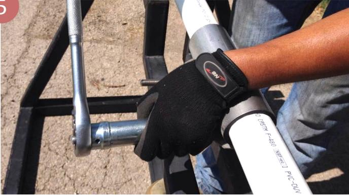
Evenly tighten the bolts working from the center outward. Maintain an even gap between bolt lugs when installing multi-panel repair clamps.
