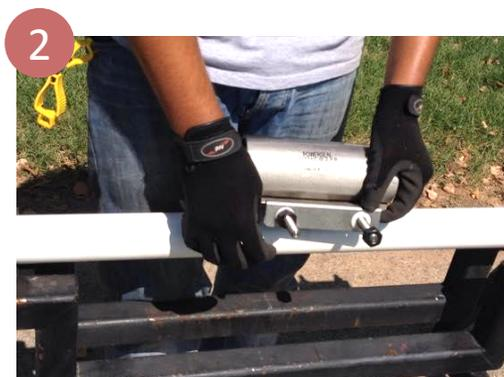
2 Loosen nuts to the end of the stud bolt, and place the clamp around the pipe centered over the break or damage area with the gasket flap at the top.
