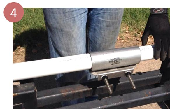
4 Rotate the clamp to flatten the tapered-end of the gasket, and position the bolts and nuts for convenient tightening. Check the reference mark (if used).
