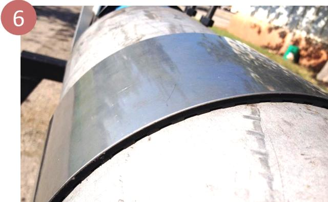
Allow the gasket to fully compress, and recheck the bolt tightness according to the recommended torque (30-35 ft-lb). It is important to re-torque bolts once clamp is already installed.
