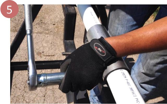
Evenly tighten the bolts working from the center outward and maintain an even gap between bolt lugs to make the gasket evenly compressed. If clamp is multi-panels keep an even gap between lugs.
