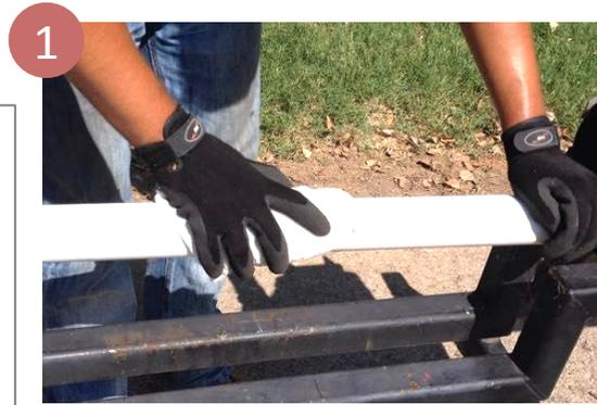
1 Thoroughly clean the pipe surface, and inspect the area where the collar leak will be installed for flaws, i.e., gouges, protrusions, excessive corrosion, etc.
