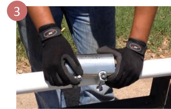
3 Place the clamp and the gasket around the pipe centered over the break or damaged area. Once in position, close the ends bringing the bolt head toward the hook of the lug, making both ends to be parallel to each other. Engage all bolt head on the hook of the lugs
