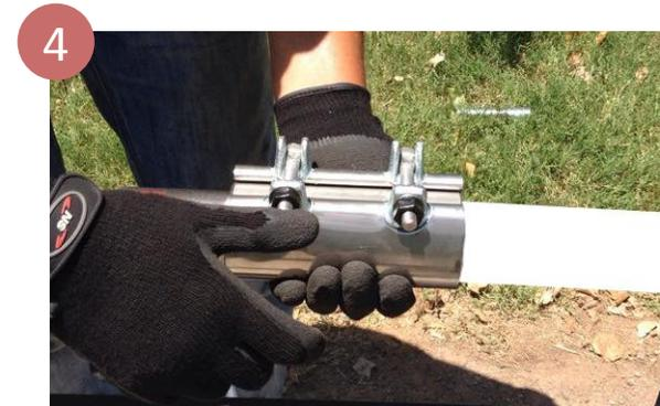
4 Smoothly rotate the Clamp and position the bolts and nuts for convenient tightening. Check the reference mark if used.
