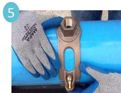
5 Loosen nut(s) to the end of the bolt and install saddle Back (s), around the pipe and through the saddle body bolt opening.
