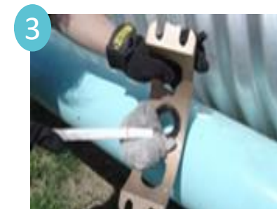
3 Lubricate pipe and face of gasket with soap and water or other suitable liquid. For cold weather lubrication, ethylene glycol can be added to the soap solution to prevent freezing.
