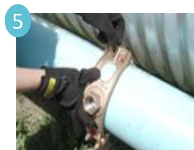
5 Loosen nut(s) to the end of the bolt and install saddle Back/Straps (s), around the pipe and through the saddle body bolt opening.
