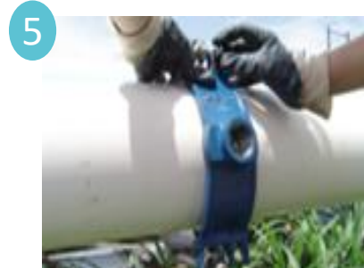
5 Loosen nuts to the end of the bolt and install saddle Back (s), around the pipe and through the saddle body bolt opening.
