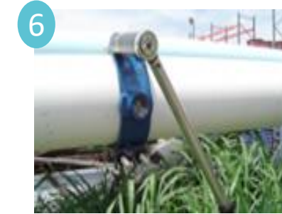
6 Tighten nuts evenly per the specifications below until saddle body conforms to pipe.
