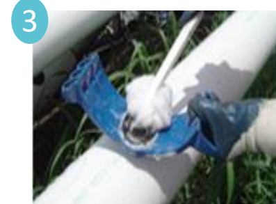
3 Lubricate pipe and face of gasket with soap and water. For cold weather lubrication, ethylene glycol can be added to the soap solution to prevent freezing.
