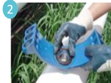
2 Confirm the PowerSeal Twin Seal saddle gasket is in the proper position in the saddle body.
