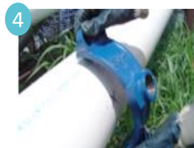
4 Position the saddle Top on the pipe in the location where it is to be tapped. Rotation of the saddle should be avoided at all times.
