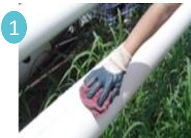
1 Clean outside of pipe thoroughly, particularly in area where Twin Seal gasket will compress.
