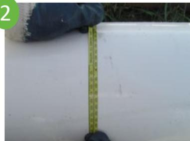
Check the main outside diameter (OD) and confirm that it falls within the tapping sleeve pipe OD range.
