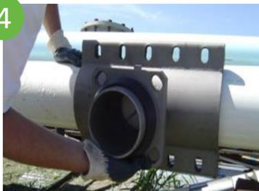
Position flanged (or Mechanical joint) half of sleeve on pipe making sure outlet is properly aligned with branch-line to be connected. Never position so that rotation of sleeve is required.
