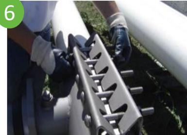
Install bolts, washers and nuts. Tighten maintaining an even gap distance between the bolt lugs on both sides of the sleeve. Nuts must be tighten in the order shown in the image.
