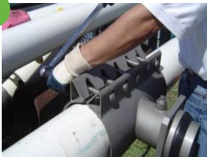
Begin tightening bolts in sequence, beginning at the ends of the sleeve and alternating on both sides. The gap between the two halves must be of equal distance when sleeve is fully tightened.
