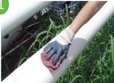
Thoroughly clean the pipe so surface is smooth and free of dirt and other debris.
