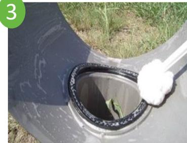
Lubricate pipe, O-Ring or hydro twin gasket with soap/water solution. Do not use grease or pipe lubricant.
