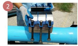
Loosen nuts to the end of the stud bolt, and place the clamp around the pipe centered over the break or damage area with the gasket flap at the top.
