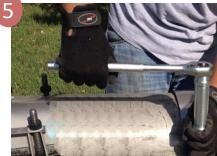
Evenly tighten the studs working from the center outward. Maintain an equal gap between the ends of all panels when installing multi-panel repair clamps.
