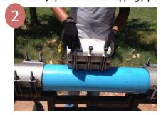
Loosen nuts to the end of the stud, place the clamp around the pipe centered over the break or damage area with the gasket flap at the top.
