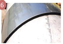
Allow the gasket to fully compress and recheck the studs tightness. It is important to re-torque Tapped Repair Clamps when used as a "hot tap" saddle after the tap has been made.
