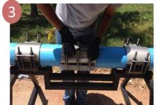
Tuck the gasket flap in place, close the fingers studs, engage the centermost stud(s) and finger tighten. NOTE: The clamp can be assembled beside the break and slid over the damaged area if the pipe surface and gasket have been properly lubricated.
