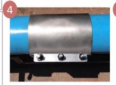
Rotate the clamp to flatten the tapered-end of the gasket and position the bolts and nuts for convenient tightening. Check the reference mark (if used).
