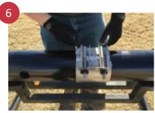
Allow the gasket to fully compress, and recheck the bolt tightness. It is important to re-torque Tapped Repair clamps when used as a "hot tap" saddle after the tap has been made. Torque the bolts as evenly as possible:
