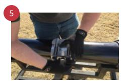
Evenly tighten the bolts working from the center outward. Maintain an even gap between bolt lugs when installing multipanel repair clamps.
