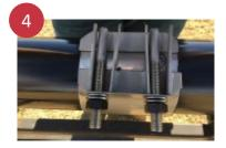
Rotate the clamp to flatten the tapered-end of the gasket, and position the bolts and nuts for convenient tightening. Check the reference mark (if used).
