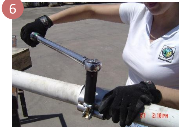
Tighten nuts until clamp is tight or leak is stopped (approximately 50ft-lb of torque).
