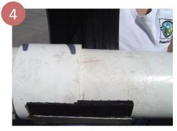
Position the step gasket making sure the thicker part of the gasket goes on the smaller diameter (pipe) and the thinner part goes on the larger diameter (Collar or Bell).
