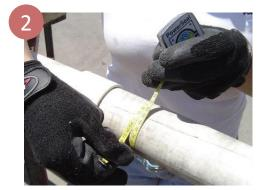
Check both outside diameters (OD) and make sure you have the proper step gasket collar leak.
