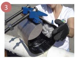
Loosen the nut to the end of the bolt and open the clamp. Do not disassemble. Lubricate pipe and gasket with soap/water solution.
