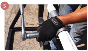
Evenly tighten the bolts working from the center outward. Maintain an even gap between bolt lugs when installing multipanel repair clamps.
