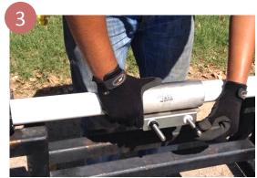
Tuck the gasket flap in place, close the bolt lug, engage the centermost bolt(s) and finger tighten. NOTE: using the palm of your hand, squeeze the end of the clamp fingers and the top of the stud lug to bring stud bolt and fingers parallel.
