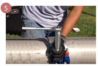
Evenly tighten the bolts working from the center outward and maintain an even gap between bolt lugs to make the gasket evenly compressed. If clamp is multi-panels keep an even gap between lugs.
