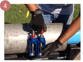
Smoothly rotate the Clamp and position the bolts and nuts for convenient tightening. Check the reference mark if used.
