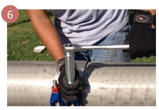
Allow the gasket to fully compress, and recheck the bolt tightness according to the recommended torque (35-70 ft-lb). It is important to re-torque bolts once clamp is already installed.
