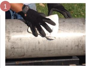
Thoroughly clean the pipe where the clamp will be installed.
