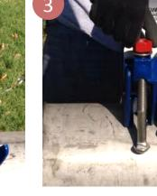
Once the Patch Clamp is in position, close the ends bringing the bolt head toward the hook of the lug, making both ends to be parallel to each other. Engage all bolt head on the hook of the lugs. Note: Clamp can be assembled aside of the break and then slid over the damaged area only if pipe surface and gasket have been properly lubricated.
