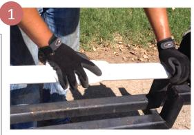
Thoroughly clean the pipe surface, and inspect the area where the collar leak will be installed for flaws, i.e., gouges, protrusions, excessive corrosion, etc.
