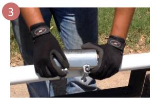
Place the clamp and the gasket around the pipe centered over the break or damaged area. Once in position, close the ends bringing the bolt head toward the hook of the lug, making both ends to be parallel to each other. Engage all bolt head on the hook of the lugs
