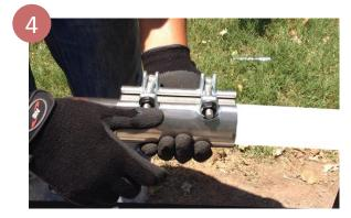
Smoothly rotate the Clamp and position the bolts and nuts for convenient tightening. Check the reference mark if used.
