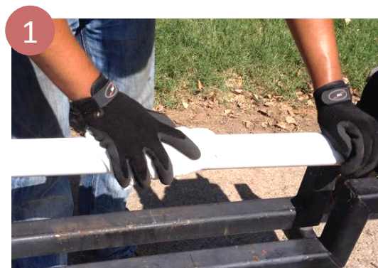
1 Thoroughly clean the pipe where the clamp will be installed.
