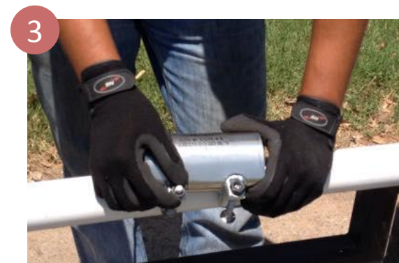
3 Loosen nuts to the end of the stud bolt, and place the clamp around the pipe over the gasket and center it over the break or damaged area.
