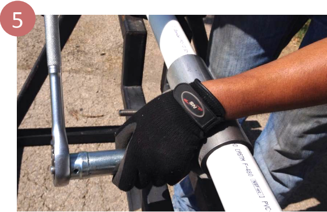
Evenly tighten the bolts working from the center outward. Maintain an even gap between bolt lugs when installing multi-panel repair clamps.
