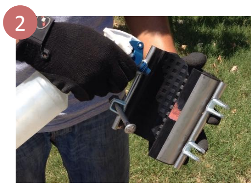
2 Remove the gasket from the clamp and wrap it around the pipe.
