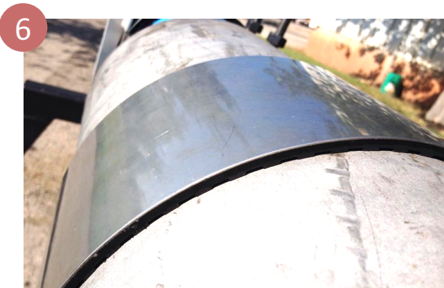
Allow the gasket to fully compress, and recheck the bolt tightness according to the recommended torque (30-35 ft-lb). It is important to re-torque bolts once clamp is already installed.
