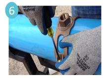
Tighten securely to a minimum of 5 ft.-lbs. of torque - which will snug the brass casting around the pipe (*halves do not meet*) with a 10" to 12" screwdriver.
