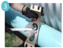
Lubricate pipe and face of gasket with soap and water or other suitable liquid. For cold weather lubrication, ethylene glycol can be added to the soap solution to prevent freezing.
