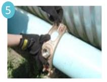
Loosen nut(s) to the end of the bolt and install saddle Back/Straps (s), around the pipe and through the saddle body bolt opening.
