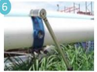
Tighten nuts evenly per the specifications below until saddle body conforms to pipe.
