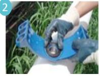
Confirm the PowerSeal Twin Seal saddle gasket is in the proper position in the saddle body.
