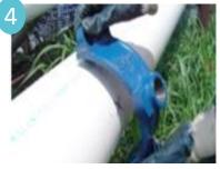
Position the saddle Top on the pipe in the location where it is to be tapped. Rotation of the saddle should be avoided at all times.
