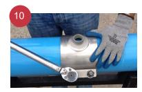
If dry tapping follow the above, but also retorque the nuts after field testing to compensate for pipe expansion.
