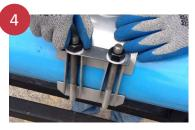
Close lug fingers and studs together by pulling the washer bar upward and snap the lip over the finger base plate. Finger tighten nuts.
