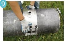
If necessary to reposition, loosen nuts prior to moving saddle and then re-torque.
