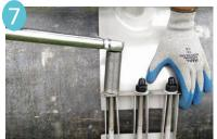
Tighten bolts in sequence, beginning at the ends of the saddle and alternating on both sides. The gap between the lugs must be of equal distance when saddle is fully tightened.
