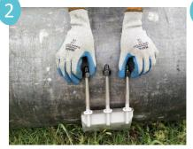
Loosen nuts until flush with top of studs.
