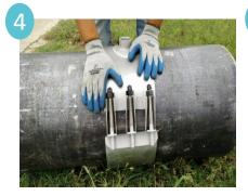
Position back panel and the top panel (outlet side) of the saddle in the desired position.
