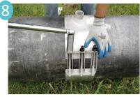
Torque nuts at 70 - 100 ft-lb to form a gasket seal. Do not over torque as it will not increase sealing ability and may cause plastic pipe failure.
