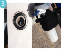
Lubrcate the O-ring with a soap solution which reduces friction and more evenly distributes clamping force. For cold weather lubrication, ethylene glycol can be added to the soap solution to prevent freezing.
