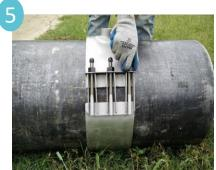
Close lug fingers and studs together by pulling the washer bar upward and lifting it over the finger baseplate. Loosely tighten nuts.
