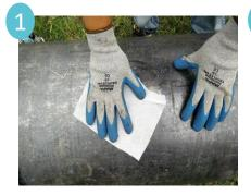
Thoroughly clean the pipe so surface is smooth and free of dirt and other debris.
