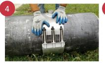
Position back panel and the top panel (outlet side) of the saddle locating the outlet in desired position.
