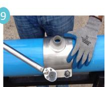
Leave each connection exposed and field pressure test prior to backfilling to assure proper installation on the pipe.
