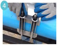
Close lug fingers and studs together by pulling the washer bar upward and snapping the lip over the finger baseplate. Loosely tighten nuts.
