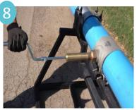
Tap through corporation stop utilizing a VegaDrill for best results on plastic pipe.
