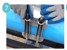
If necessary to reposition, loosen nuts prior to moving saddle and then retorque.
