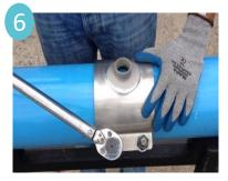
Torque nuts 50 - 70 ft/lbs to form a gasket seal. Do not over torque as it will not increase sealing ability and may cause plastic pipe failure.
