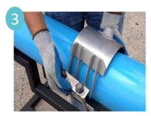
Loosen nuts until flush with top of studs, and place saddle around pipe.
