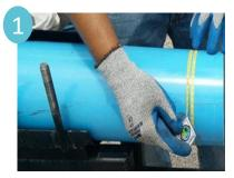
Check pipe diameter to insure that correct saddle is being installed.
