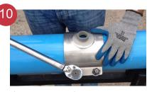
Leave each connection exposed and field pressure test prior to backfilling to assure proper installation on the pipe.
