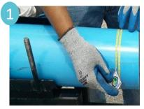
Check pipe diameter to insure that correct saddle is being installed.
