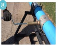
Tap through corporation stop utilizing a VegaDrill for best results on plastic pipe.
