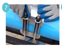
If necessary to reposition, loosen nuts prior to moving saddle and then retorque.
