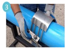
Loosen nuts until flush with top of studs, and place saddle around pipe.
