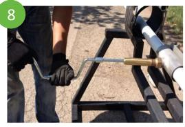
Hydrostatic pressure test, then tap through a valve using a VegaDrill for best results on plastic pipe.
