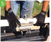
Locate and place nipple in desired position.
