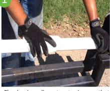
Check pipe diameter to insure that the correct fitting is being installed. Thoroughly clean the pipe surface until it is smooth and free of dirt and other debris.
