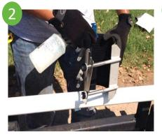
Lubricate the gasket with a soap solution. For cold weather lubrication, ethylene glycol can be added to the soap solution to prevent freezing.
