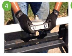
Close lug fingers and studs together by pulling the washer bar upward and snap the lip over the finger base plate. Manually tighten nuts.
