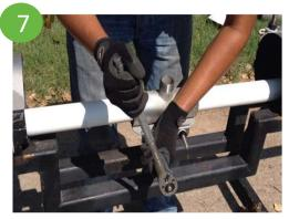
If necessary to reposition, loosen nuts prior to moving fitting and then retorque.
