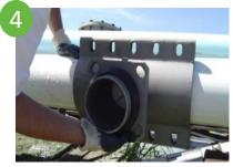
Position flanged (or Mechanical joint) half of sleeve on pipe making sure outlet is properly aligned with branch-line to be connected. Never position so that rotation of sleeve is required.
