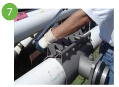
Begin tightening bolts in sequence, beginning at the ends of the sleeve and alternating on both sides. The gap between the two halves must be of equal distance when sleeve is fully tightened.
