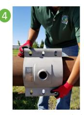
Position the outlet half of sleeve on pipe making sure is properly aligned with the line to be connected.
