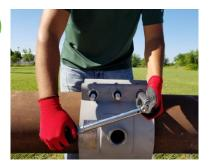
Begin tightening bolts in sequence, beginning at the ends of the sleeve and alternating on both sides. The gap between the two halves must be of equal distance when sleeve is fully tightened. Torque according the specifications. Wait approximately 5 minutes to allow the gasket to fully compress and then re-tighten bolts.
