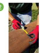
Check the main outside diameter (OD) and confirm that it falls within the tapping sleeve pipe OD range.
