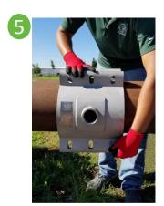
Position back half of sleeve behind the outlet half aligning bolt holes.
