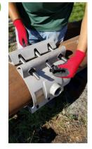
Install bolts, washers and nuts. Tighten maintaining an even gap distance between the bolt lugs on both sides of the sleeve.
