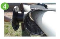
Position flanged (or MJ-Mechanical Joint) half of sleeve on pipe making sure outlet is properly aligned with branch-line to be connected. Make certain that the tapered ends of the complete circle gasket are smooth against the pipe. Never position so that rotation of sleeve is required.
