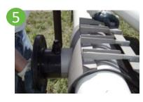
Position back half of sleeve over the tapered ends of the gasket being careful not to fold or roll the edges under themselves. Locate Bolts between fingers on the flanged half of sleeve.
