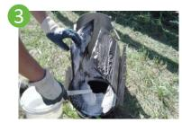
Lubricate pipe and gasket with soap/water solution. **Do not use grease or pipe lubricant.**
