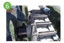
Install washer bar, delrin washer and nuts. Tighten maintaining an even gap distance between the panels on both sides of the sleeve. Nuts must be tighten in the order shown in the image.
