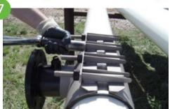
Begin tightening bolts in sequence, beginning at the center of the sleeve and alternating on both sides. The gap between the two halves must be of equal distance when sleeve is fully tightened.
