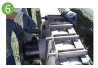
Install washer bar, spring washers and nuts. Tighten maintaining an even gap distance between the panels on both sides of the sleeve. Nuts must be tighten in the order shown in the image.
