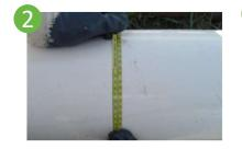
Check the main outside diameter (OD) and confirm that it falls within the tapping sleeve pipe OD range.
