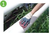
Thoroughly clean the pipe so surface is smooth and free of dirt and other debris.
