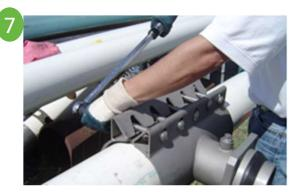
Tighten bolts in sequence, beginning at the ends of the sleeve and alternating on both sides. The gap between the two halves must be of equal distance when sleeve is fully tightened.
