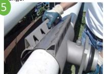
Make certain that the tapered ends of the complete circle gasket are smooth against the pipe, and position back half of sleeve over the tapered ends of the gasket being careful not to fold or roll the edges under themselves.
