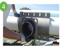
Position flanged (or MJ-Mechanical Joint) half of sleeve on pipe making sure outlet is properly aligned with branch-line to be connected. Make certain that the tapered ends of the complete circle gasket are smooth against the pipe. **Never position so that rotation of sleeve is required**.
