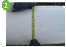
Check the main outside diameter (OD) and confirm that it falls within the tapping sleeve pipe OD range.
