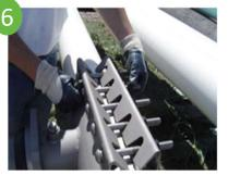
Install bolts, washers and nuts. Tighten maintaining an even gap distance between the bolt lugs on both sides of the sleeve; i.e. 25 ftlb increments. Nuts must be tighten in the order shown in the image.
