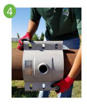
Position the outlet half of sleeve on pipe making sure is properly aligned with the line to be connected.
