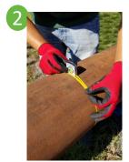
Check the main outside diameter (OD) and confirm that it falls within the tapping sleeve pipe OD range.
