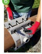
Install bolts. washers Tighten and nuts. maintaining an even gap distance between the bolt lugs on both sides of the sleeve.
