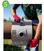
Position back half of sleeve behind the outlet half aligning bolt holes.
