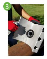
Loosen bolts and nuts. Lubricate pipe and O-Ring gasket with soap/water solution. Do not use grease or pipe lubricant.
