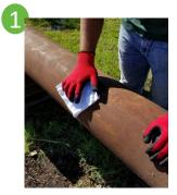
Thoroughly clean the pipe so surface is smooth and free of dirt and other debris.
