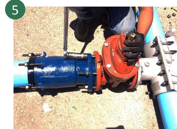
5 Evenly tighten MJ bolts in a radial pattern and then proceed to evenly tighten gland bolts to the suggested torques.
