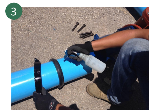
3 Lubricate pipe end and coupling gasket with a soapy solution.
