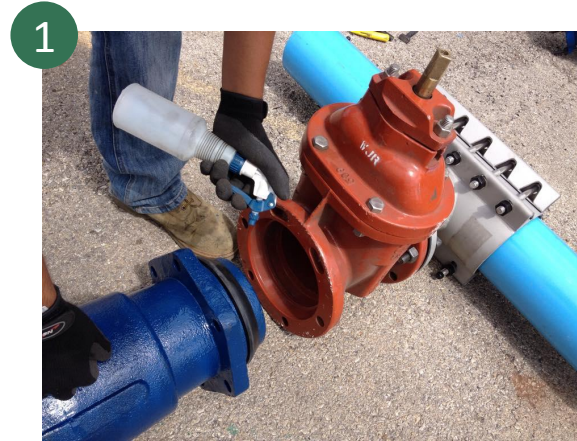
1 Lubricate MJ gasket and connect the MJ adapter to MJ Valve or fitting.
