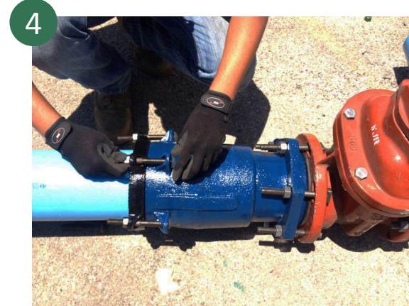
4 Hand tighten gland bolts and stab plain-end pipe into coupling.
