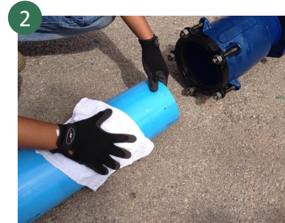
2 Thoroughly clean the pipe end where the cutting-In sleeve will be installed.
