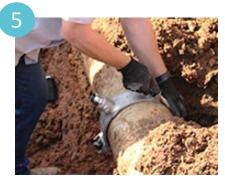
Loosen nuts to the end of the bolt and install strap (s), around the pipe and through the saddle body bolt opening.
