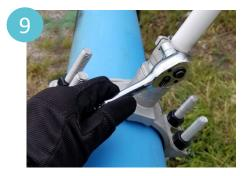
Once the gasket begins to compress, tighten the pack joint nut 1 to 1-1/2 rotations. DO NOT USE A PIPE WRENCH. We recommend using a flat adjustable wrench. Make sure to securely tighten the clamp screw with a socket to avoid a pipe/tubing blowout.
