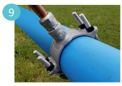
Start to tighten the PowerJoint nut. Once the gasket begins to compress, tighten the PowerJoint nut all the way to the bottom. DO NOT USE A PIPE WRENCH. We recommend using a flat adjustable wrench.
