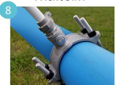
Re-install the pack joint nut. Insert pipe/tubing into the fitting until it has passed the seal gasket. Ensure the pipe/tubing diameter size corresponds with the nut that is to be installed.
