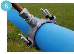
Re-install the grip joint nut. Insert pipe/tubing into the fitting until it has passed the seal gasket, then leave 1/8" space from the bottom of the corp. Ensure the pipe/tubing diameter size corresponds with the nut that is to be installed.
