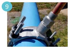
Tighten the flare joint nut all the way to the bottom, until making contact with the corp. DO NOT USE A PIPE WRENCH. We recommend using a flat adjustable wrench.
