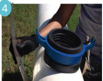
Wrap strap around pipe and slide the adjustable bolt assembly to a point which leaves most of the thread for tightening.
