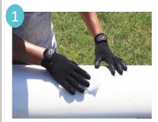
Check diameter of main and branch pipe to make sure you are using the correct size saddle gasket; also check gasket to make sure it is the size you think
