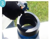
Lubricate the saddle gasket and the pipe main. Place saddle and gasket over pipe.
