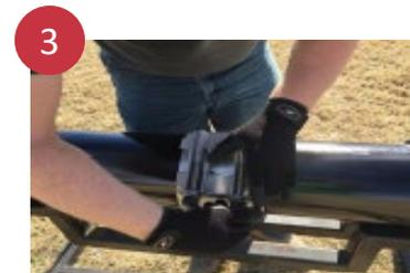
Tuck the gasket flap in place, close the bolt lug, engage the centermost bolt(s) and finger tighten. NOTE: using the palm of your hand, squeeze the end of the clamp fingers and the top of the stud lug to bring stud bolt and fingers parallel.
