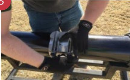
Evenly tighten the bolts working from the center outward. Maintain an even gap between bolt lugs when installing multi-panel repair clamps.
