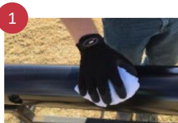
Thoroughly clean the pipe where the clamp will be installed.
