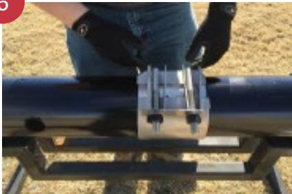
Allow the gasket to fully compress, and recheck the bolt tightness. It is important to re-torque Tapped Repair clamps when used as a "hot tap" saddle after the tap has been made. Torque the bolts as evenly as possible:
