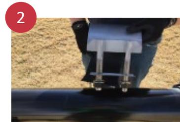
Loosen nuts to the end of the stud bolt, and place the clamp around the pipe centered over the break or damage area with the gasket flap at the top.
