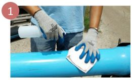
Thoroughly clean the pipe where the clamp will be installed.
