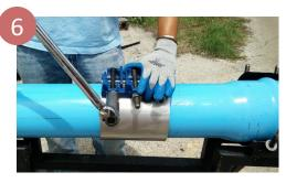
Allow the gasket to fully compress, and recheck the bolt tightness. It is important to re-torque Tapped Repair clamps when used as a "hot tap" saddle after the tap has been made. Torque the bolts as evenly as possible:
