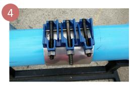
Rotate the clamp to flatten the taperedend of the gasket, and position the bolts and nuts for convenient tightening. Check the reference mark (if used).
