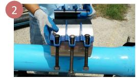
Loosen nuts to the end of the stud bolt, and place the clamp around the pipe centered over the break or damage area with the gasket flap at the top.
