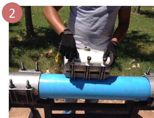
2 Loosen nuts to the end of the stud bolt, and place the clamp around the pipe centered over the break or damage area with the gasket flap at the top.
