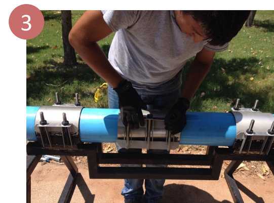
3 Tuck the gasket flap in place, close the bolt lug, engage the centermost bolt(s) and finger tighten. NOTE: The clamp can be assembled beside the break and slid over the damaged area if the pipe surface and gasket have been properly lubricated.
