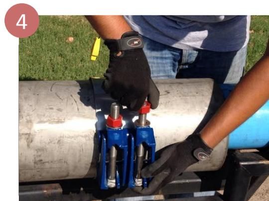
4 Smoothly rotate the Clamp and position the bolts and nuts for convenient tightening. Check the reference mark if used.
