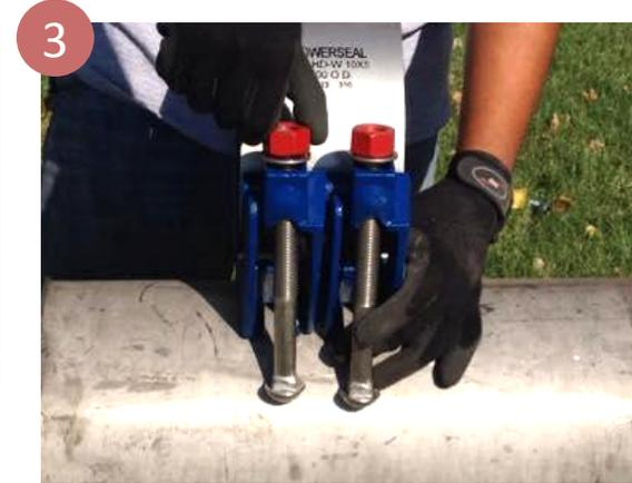
3 Once the Patch Clamp is in position, close the ends bringing the bolt head toward the hook of the lug, making both ends to be parallel to each other. Engage all bolt head on the hook of the lugs. Note: Clamp can be assembled aside of the break and then slid over the damaged area only if pipe surface and gasket have been properly lubricated.
