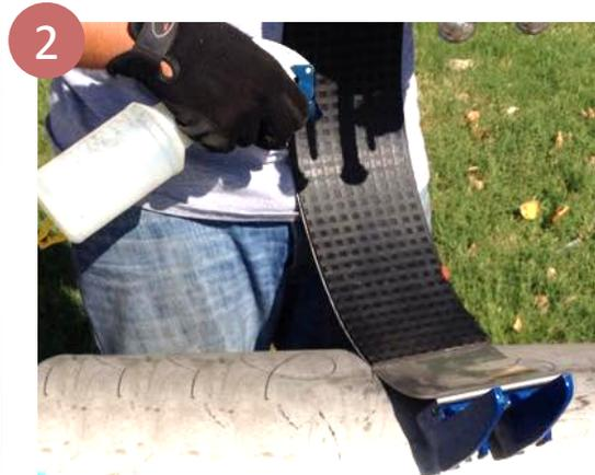
2 Loosen nuts to the end of the stud bolt, and place the clamp around the pipe centered over the break or damage area.
