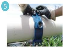
Loosen nuts to the end of the bolt and install saddle Back (s), around the pipe and through the saddle body bolt opening.
