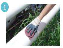
Clean outside of pipe thoroughly, particularly in area where Twin Seal gasket will compress.
