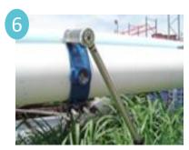
Tighten nuts evenly per the specifications below until saddle body conforms to pipe.
