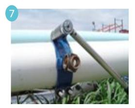
To ensure proper seal of the gasket, the corporation stop or other fittings should be connected to the saddle prior to final tightening. Always re-tighten after installation of the valve or service.
