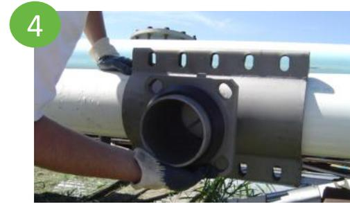
4 Position flanged (or Mechanical joint) half of sleeve on pipe making sure outlet is properly aligned with branch-line to be connected. Never position so that rotation of sleeve is required.
