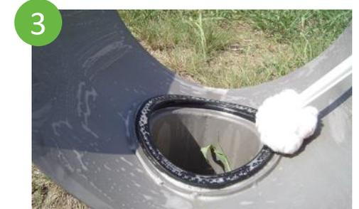
3 Lubricate pipe and hydro twin gasket with soap/water solution. Do not use grease or pipe lubricant.
