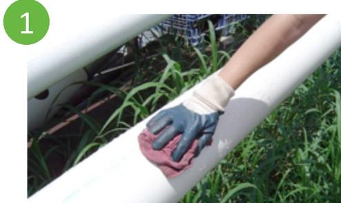
1 Thoroughly clean the pipe so surface is smooth and free of dirt and other debris.
