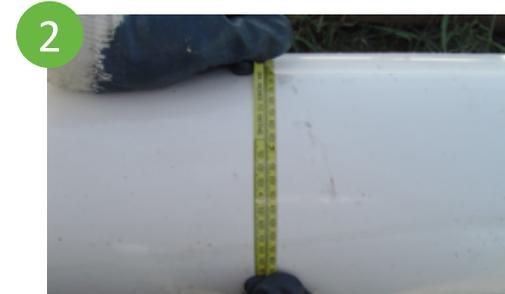
2 Check the main outside diameter (OD) and confirm that it falls within the tapping sleeve pipe OD range.
