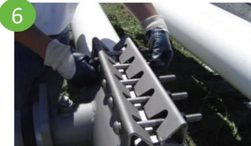
Install bolts, washers and nuts. Tighten maintaining an even gap distance between the bolt lugs on both sides of the sleeve.
