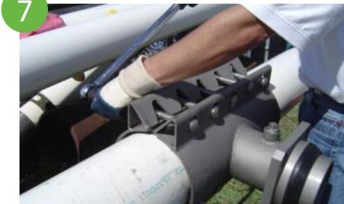
Begin tightening bolts in sequence, beginning at the ends of the sleeve and alternating on both sides. The gap between the two halves must be of equal distance when sleeve is fully tightened.
