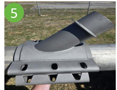
5 Position back half of wye behind the top half.
