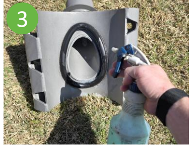
3 Lubricate pipe, O-Ring or hydro twin gasket with soap/water solution. Do not use grease or pipe lubricant.
