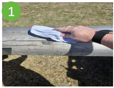
1 Thoroughly clean the pipe so surface is smooth and free of dirt and other debris.
