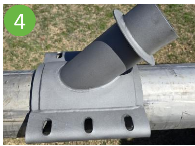
4 Position the top half of wye on pipe making sure outlet is properly aligned with branch-line to be connected. Never position so that rotation of wye is required.
