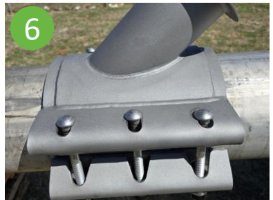
6 Install bolts, washers and nuts. Tighten maintaining an even gap distance between the bolt lugs on both sides of the wye. Nuts must be tighten in the order shown in the image.
