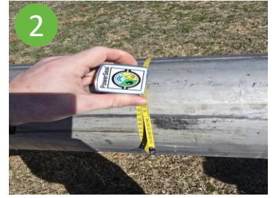
2 Check the main outside diameter (OD) and confirm that it falls within the tapping wye pipe OD range.
