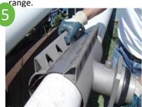
Make certain that the tapered ends of the complete circle gasket are smooth against the pipe, and position back half of sleeve over the tapered ends of the gasket being careful not to fold or roll the edges under themselves.
