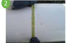
Check the main outside diameter (OD) and confirm that it falls within the tapping sleeve pipe OD cange.
