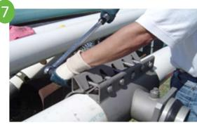
Tighten bolts in sequence, beginning at the ends of the sleeve and alternating on both sides. The gap between the two halves must be of equal distance when sleeve is fully tightened.
