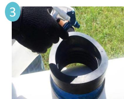
3 Lubricate the saddle gasket and the pipe main. Place saddle and gasket over pipe.
