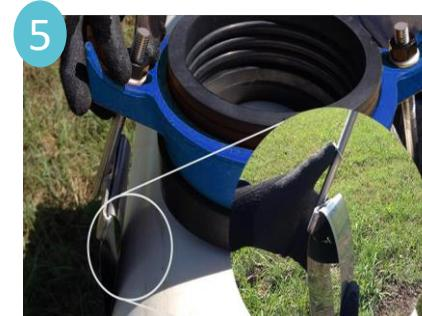
5 Fold strap back against itself, placing free end between strap and pipe. (On small pipe, it may be necessary to fold loose end twice).
