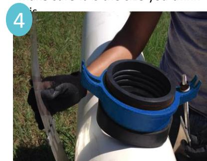
4 Wrap strap around pipe and slide the adjustable bolt assembly to a point which leaves most of the thread for tightening.
