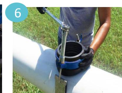
6 Tighten nuts evenly, alternating between them until appropriate torque is reached (see below). Significant flattening of PVC pipe indicates overtightening. In all cases wait 10 minutes and retorqued.
